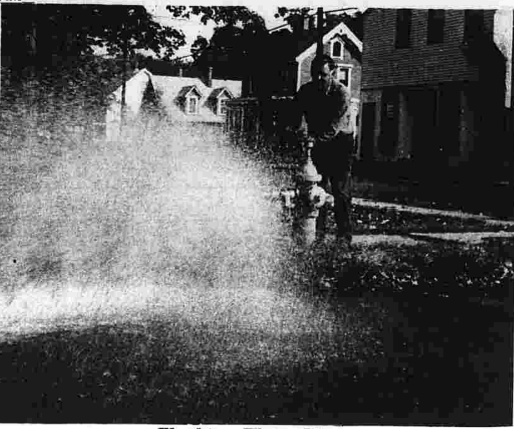
Flushing Water Line A blast of water sprays forth as George and Pina streets intersection. (Herald photo)
